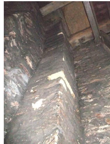
Figure 2 Flue from the second floor to the roof
