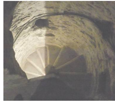
Figure 1 Stairs inside the tower
