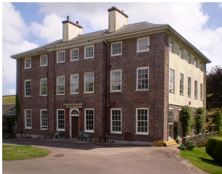
Nethway front entrance
